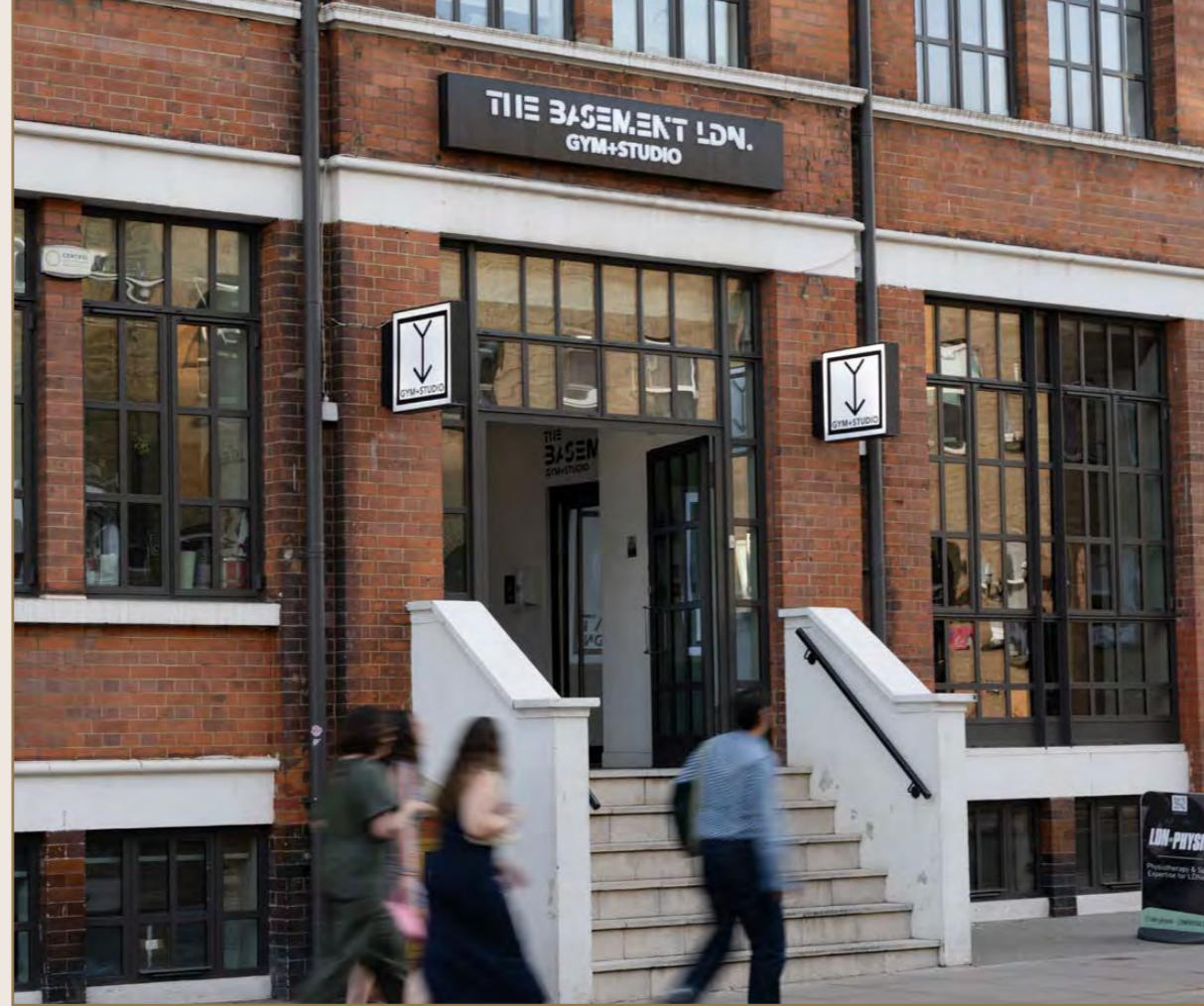
The Basement LDN Gym + Studio
